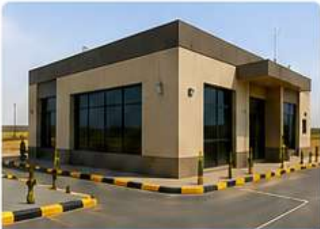
SECURITY CONTROL CENTRE
