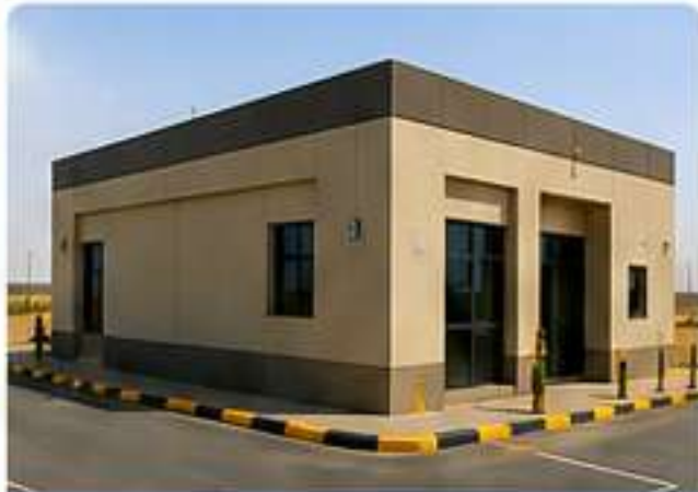
X-RAY INSPECTION BUILDING
