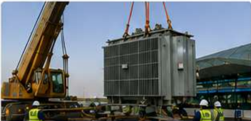
TRANSFORMER LIFTING & POSITIONING
