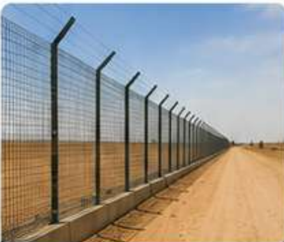
COMPLETED PERIMETER FENCE
