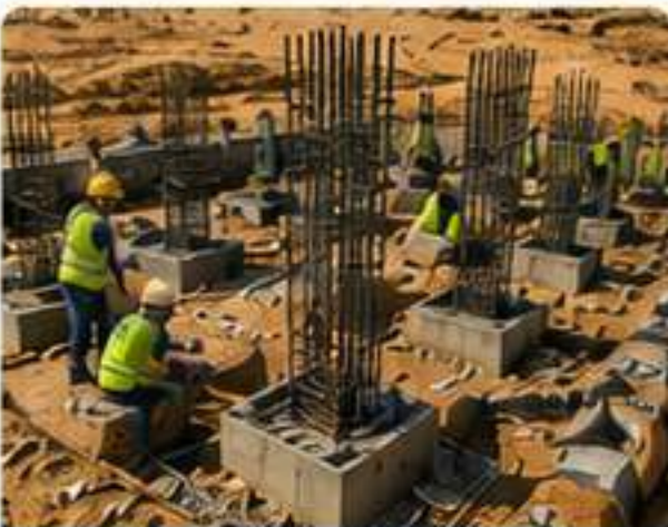
CIVIL STRUCTURAL WORKS
