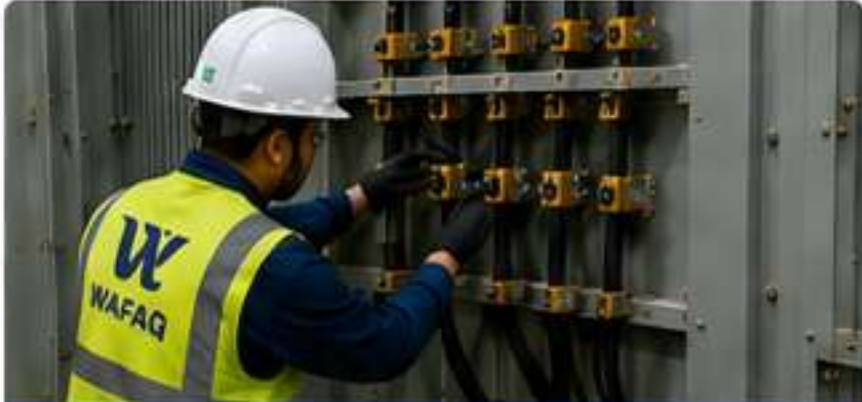
ELECTRICAL CONNECTION WORKS
