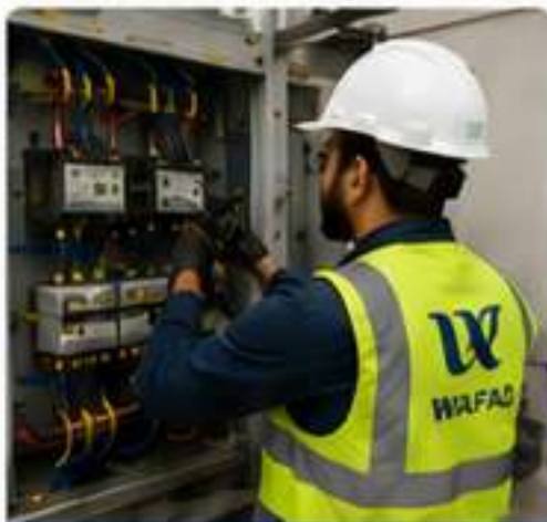
CABLE TERMINATION WORKS
