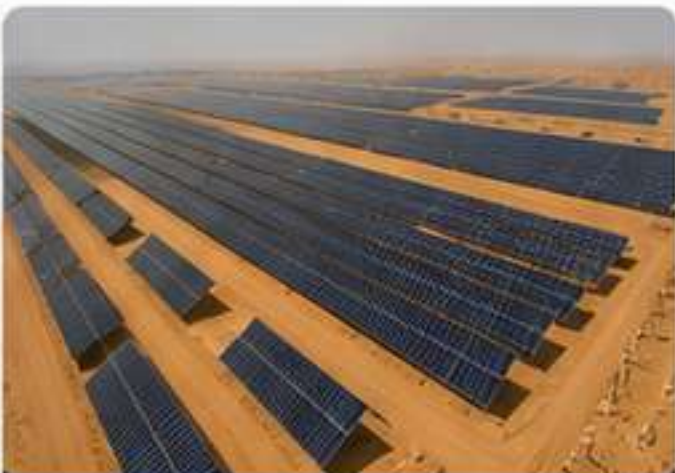
PROJECT SITE OVERVIEW
