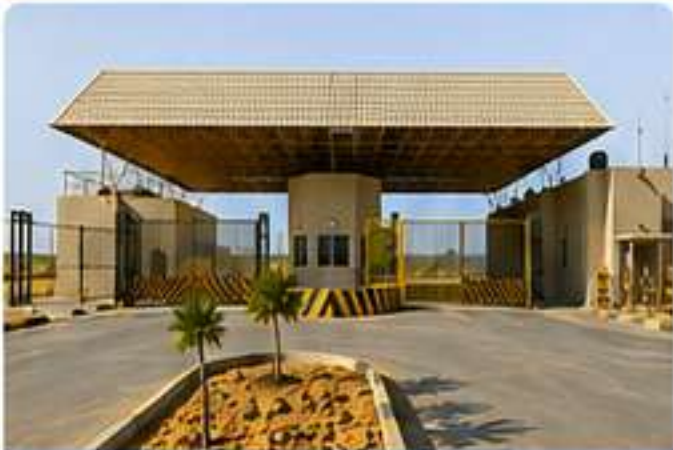
MAIN ENTRANCE & GUARD HOUSE
