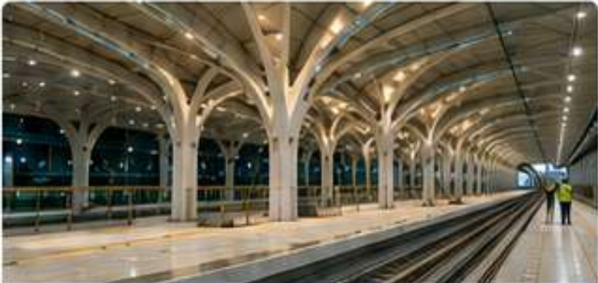
RIYADH METRO STATION INFRASTRUCTURE
