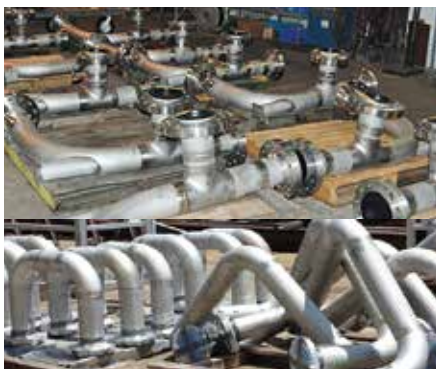
Pipe Spool Fabrication and Installation
